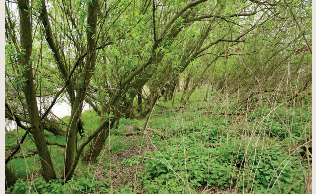
Example of an older willow mattress (no maintenance) on the Weser – Stolzenau (S. Knopp, on behalf of BfG)
